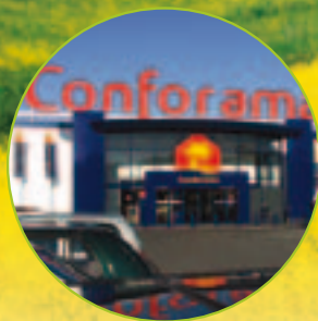
CONFORAMA Creil France
